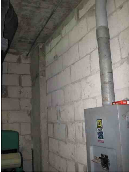
CBS wall construction
