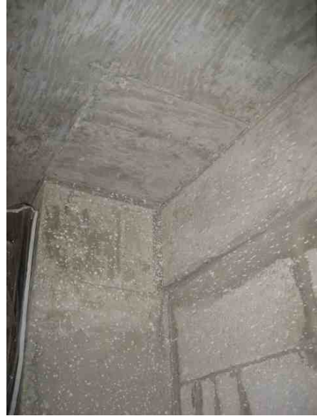
poured concrete floor & roof decks
