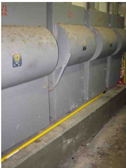
transformer vault (un-finished)
