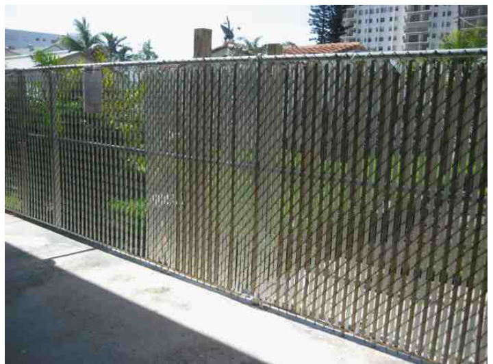
chain link fencing
