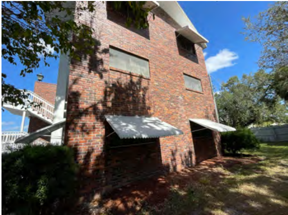
GENERAL VIEW OF BUILDING EXTERIOR FINISHES
