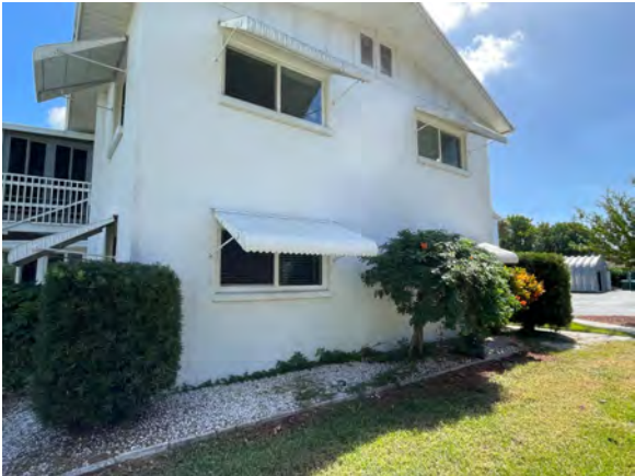
GENERAL VIEW OF BUILDING EXTERIOR FINISHES
