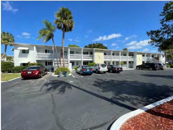
GENERAL VIEW OF PROPERTY
