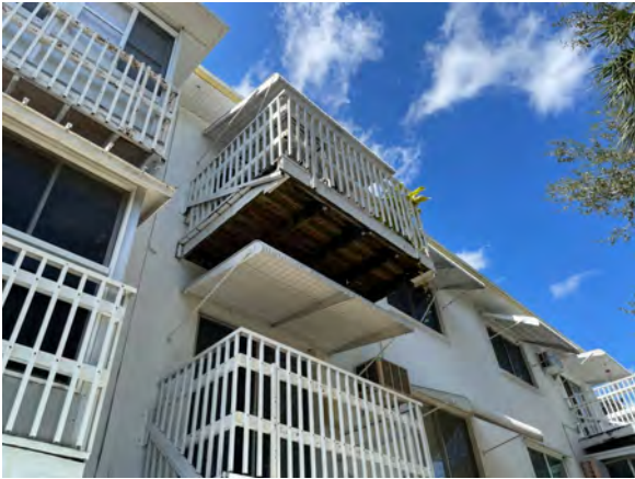
VIEW OF TYPICAL BALCONY
